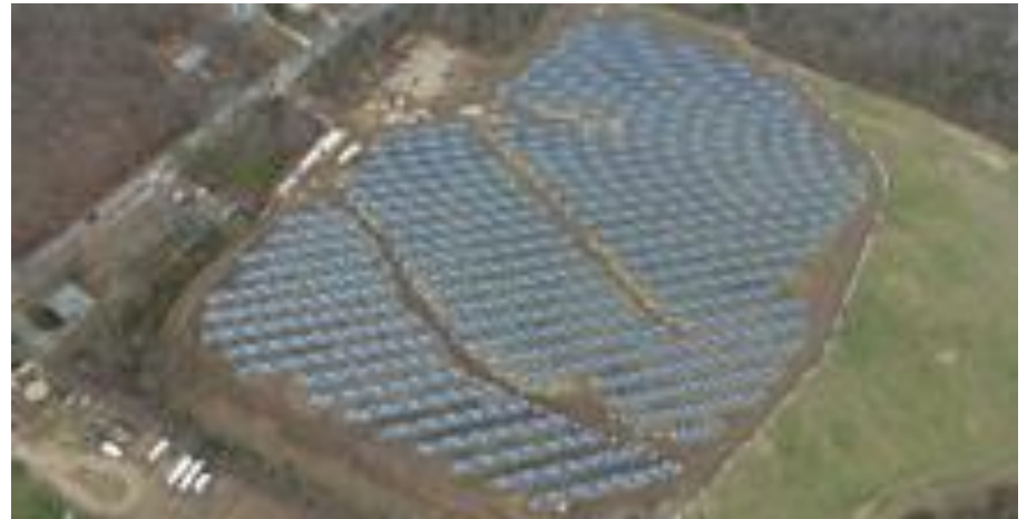
AC Power's 3.7 MWdc solar project in Gloucester Township
